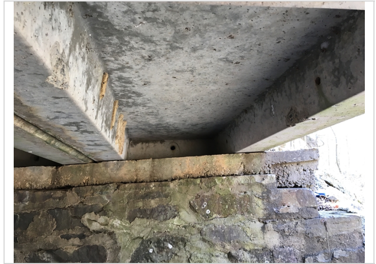
Span #1 channel unit #1 has a couple very minor spalls, this is typical in a few areas of channel units throughout both spans.
