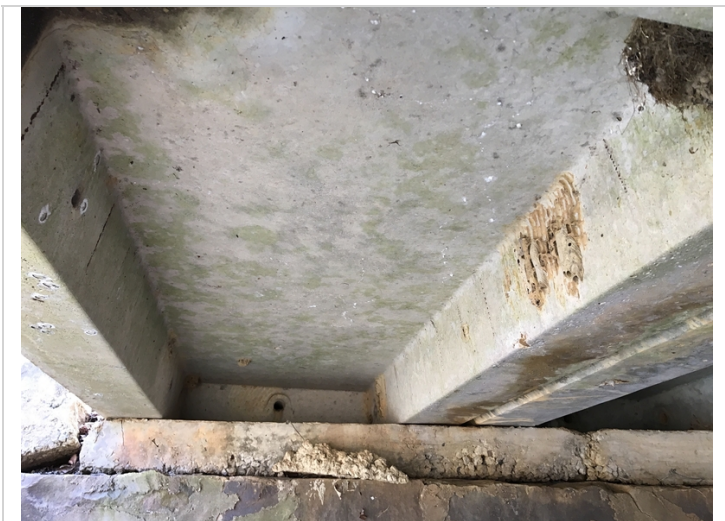
Span #1, channel unit #6 has some minor efflorescence in the soffit area.
