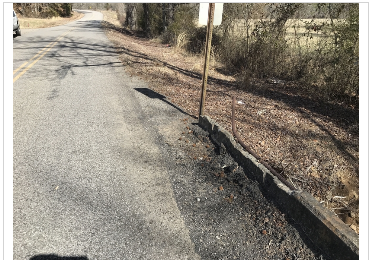
End of bridge on the right (east) side curb has approximately 8 ft. of moderate spalling with exposed rebar that is bent outward.
