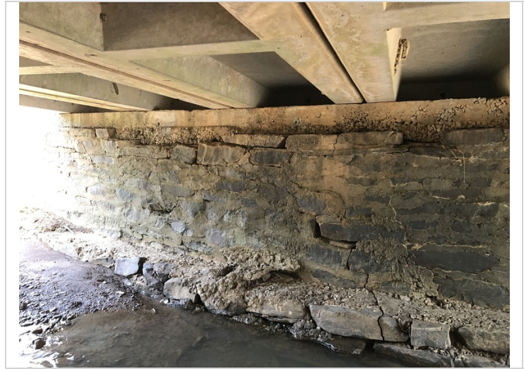
Abutment #3 has cracks in the mortar joints, has missing mortar in some joints and missing masonry stones in a few areas.
