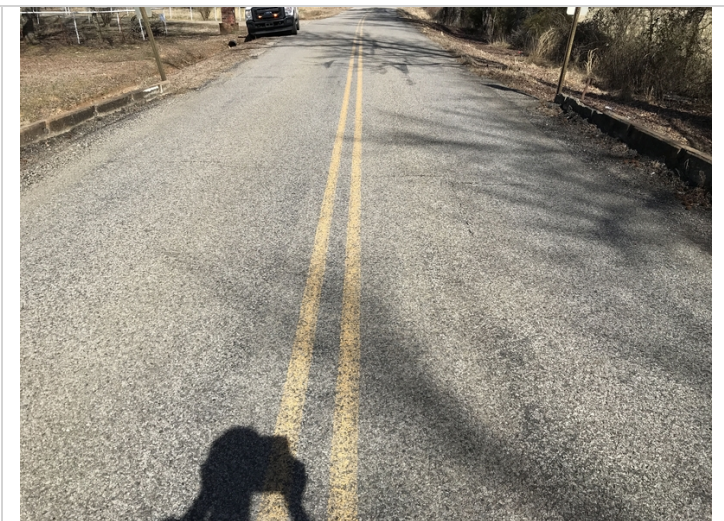
Wearing surface has a few minor cracks in places.
