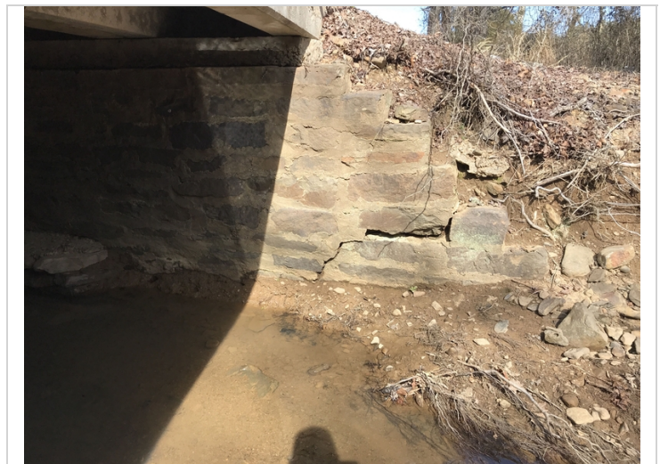
Abutment #3 right end has a large crack in the mortar joints.
