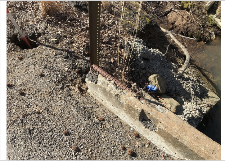
Beginning of the bridge left side curb has moderate spalling with exposed rebar.
