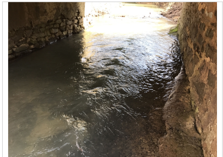
Insignificant scour in span #1, no undermining.
