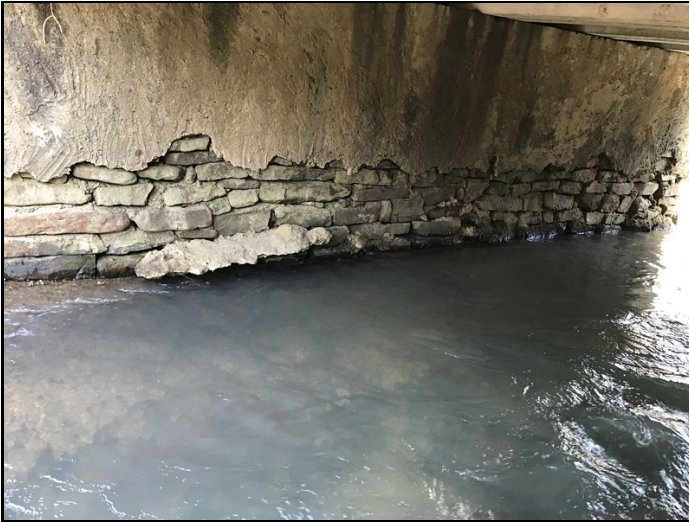
Pier #2 back side is missing grout in all the lower section of the pier wall, this is typical on the ahead side.
