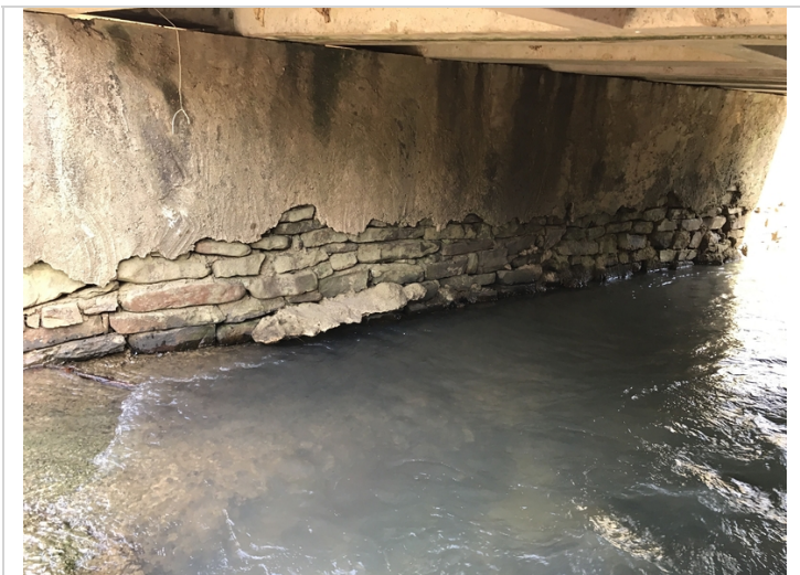
Pier #2 back side is missing grout in all the lower section of the pier wall, this is typical on the ahead side.
