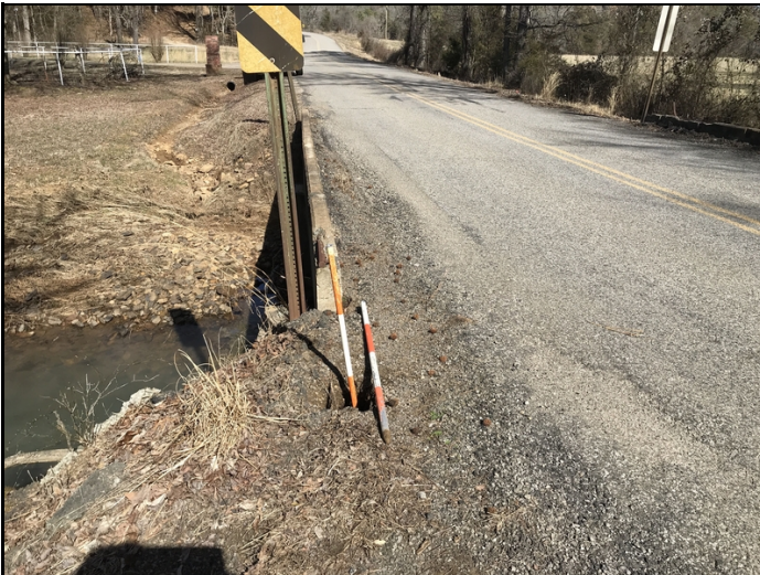
Beginning of the bridge (south end) has some moderate erosion that has created a hole approximately 2 ft. deep by 2 ft. across on the west side.
