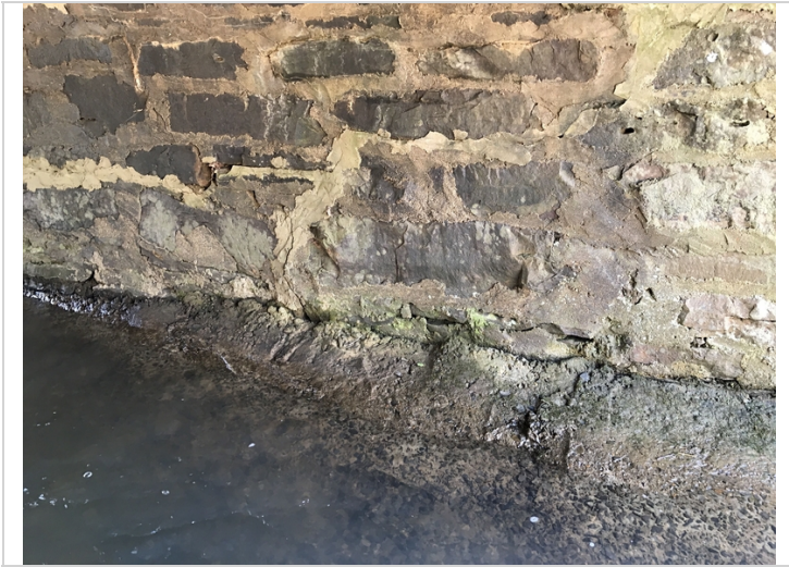
Abutment #1 has some minor to moderate cracks in the mortar joints in a few places.
