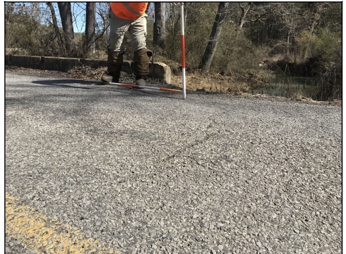
There is approximately 2-3" of settlement on the south/east side at the beginning of the bridge.
